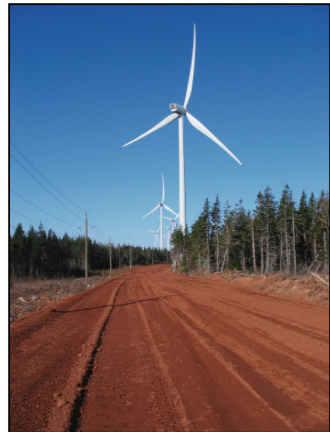
Wind farms require clearing of forest habitat for roads and infrastructure. Photo © Greg Campbell
